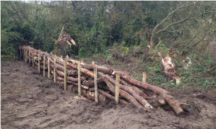
Permeable dams provide a simple, low-cost method of holding back excess flow during storm events © GWCT
